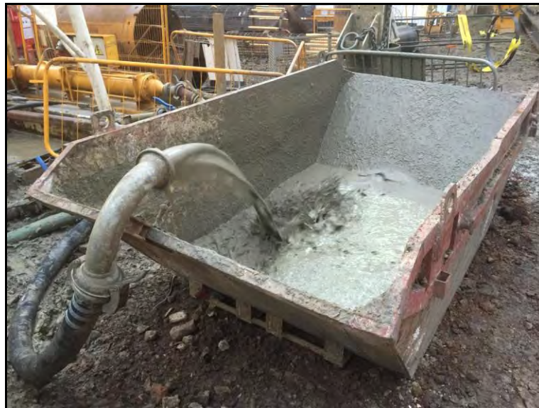
Figure 7: Skip with waste slurry
