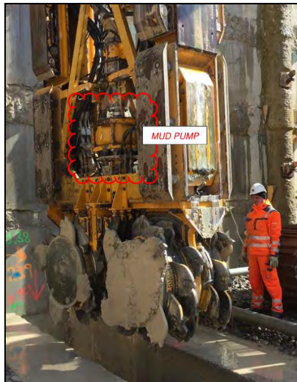
Figure 2: Cutter wheels and mud pump
