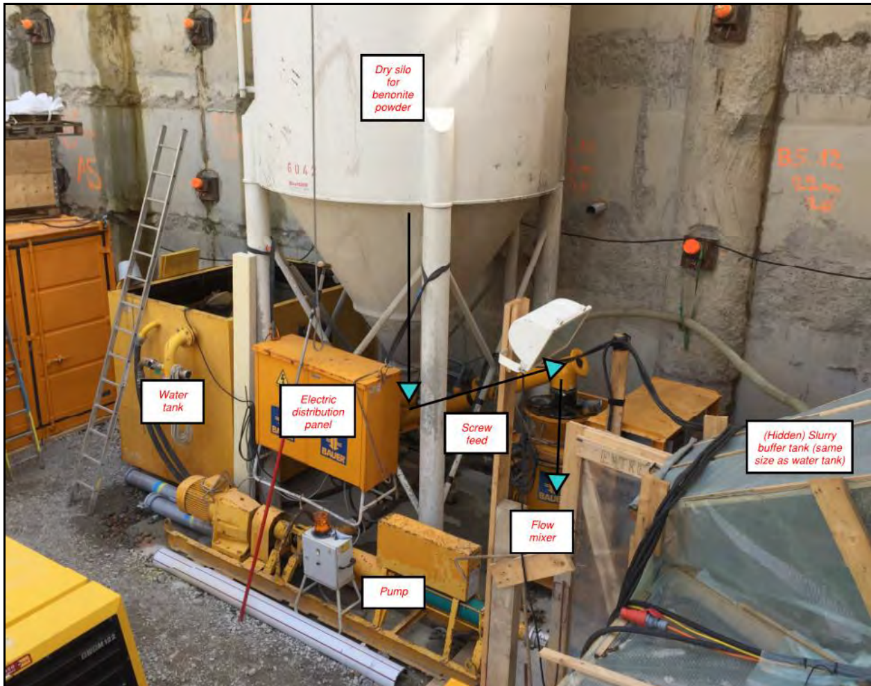
Figure 1: Typical slurry mixing setup
