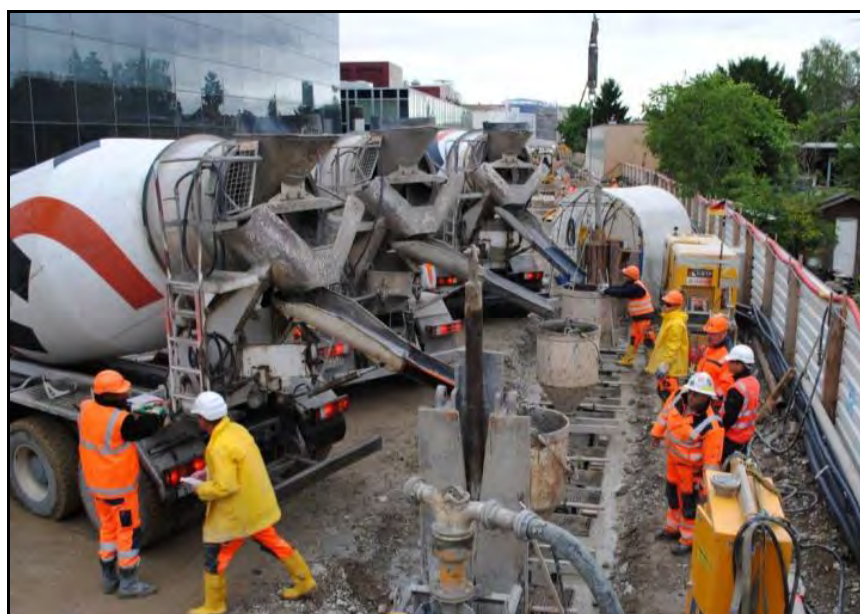
Figure 10: Photo of concrete discharge
