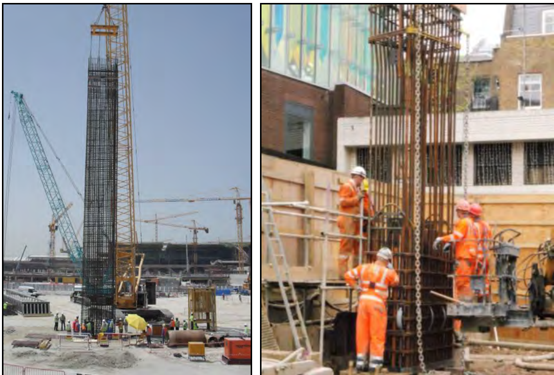
Figure 8: Photos of typical reinforcement installation
