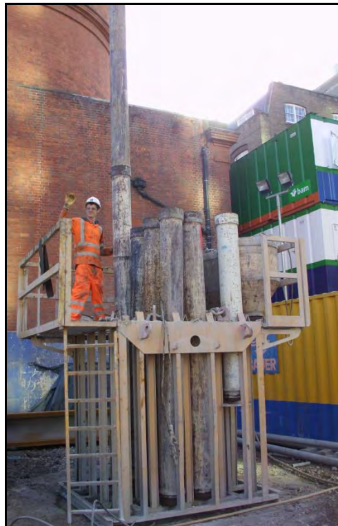
Figure 9: Photo of tremie string assembly
