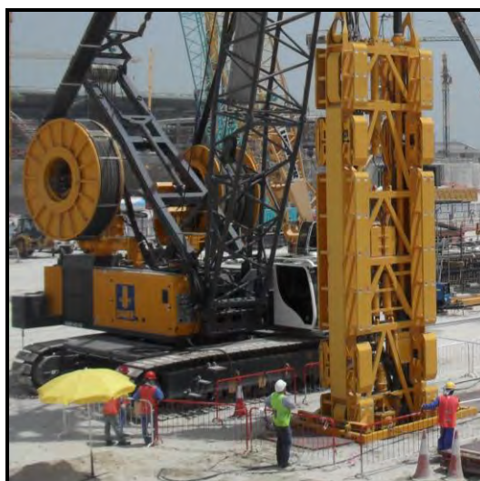
Figure 4: Cutter unit and guide frame
