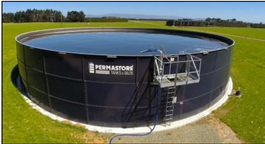
Figure 2: Photograph of typical storage tank
