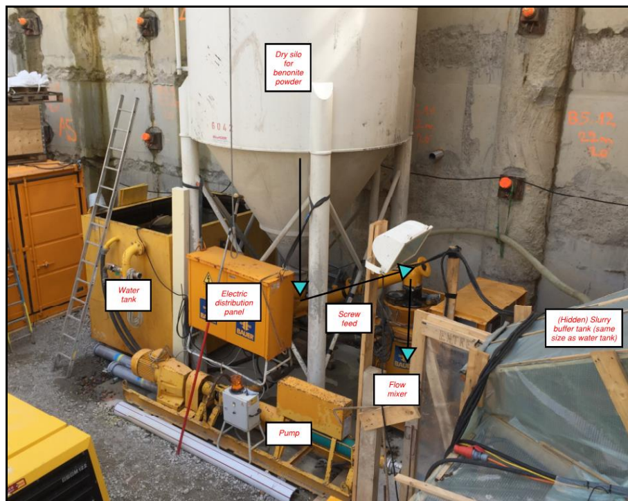
Figure 5: Typical slurry mixing setup
