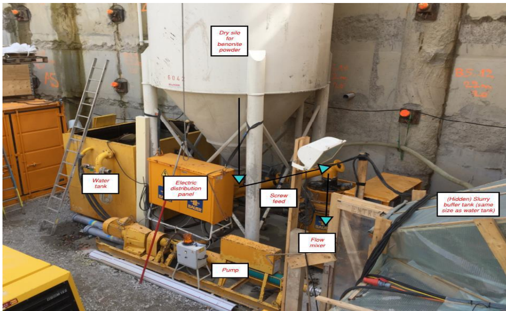
Photograph 6: Typical mixer set up
