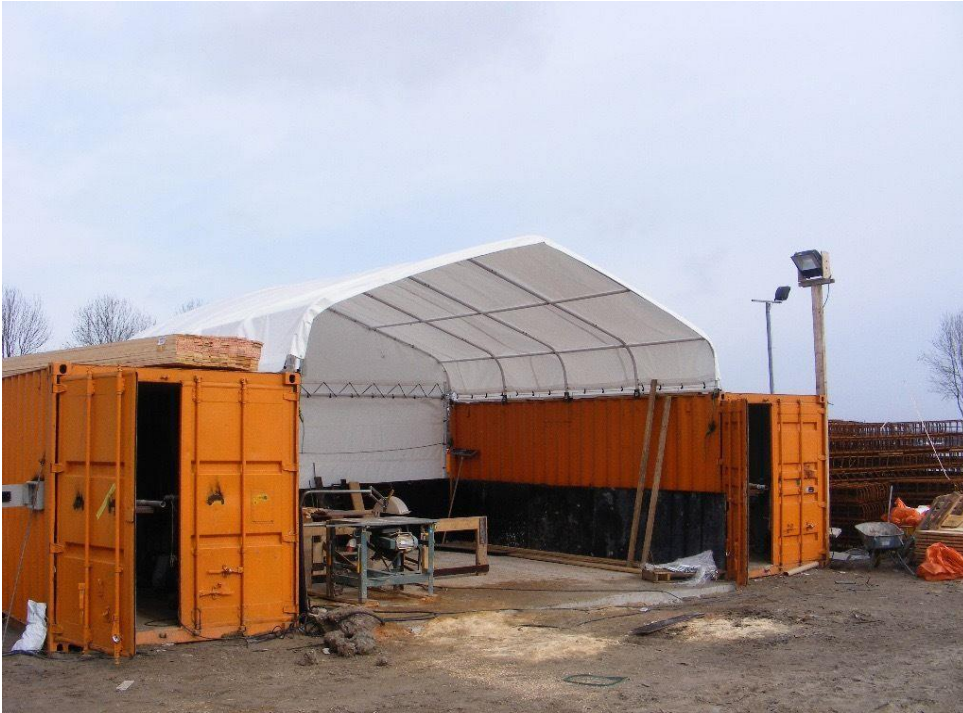
Photograph 3: Example of welding tent/shelter
