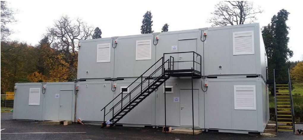
Photograph 4: Typical Welfare Facility
