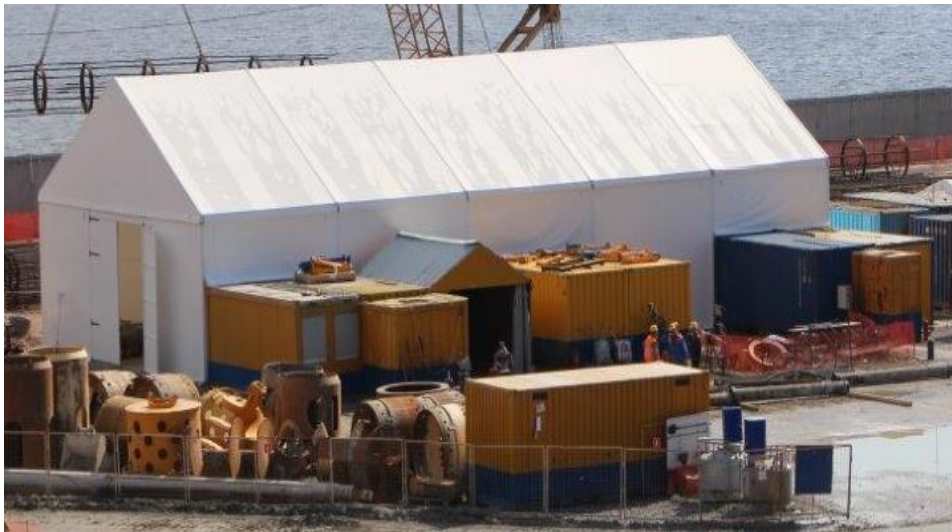
Photograph 1: Example of workshop with store containers installed to the sides
