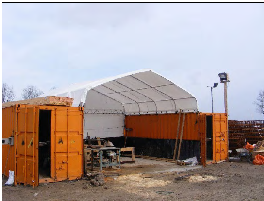
Figures 5: Example of welding tent/shelter
