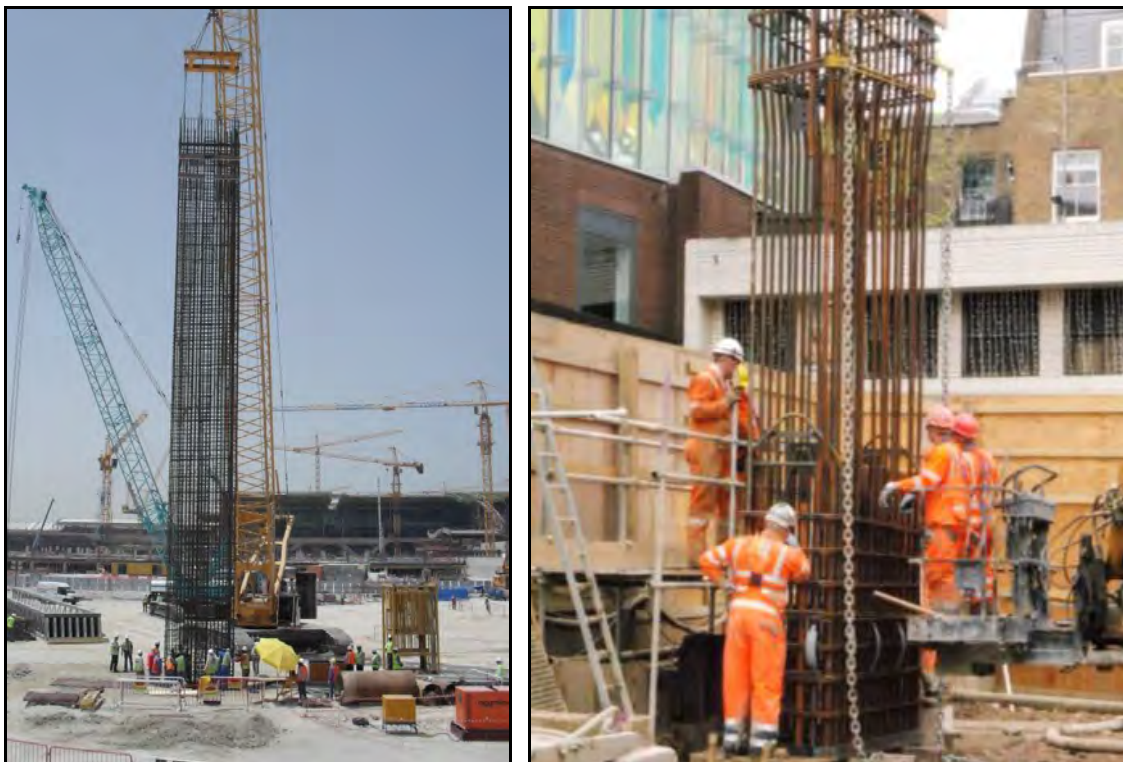
Figure 8: Photos of typical reinforcement installation
