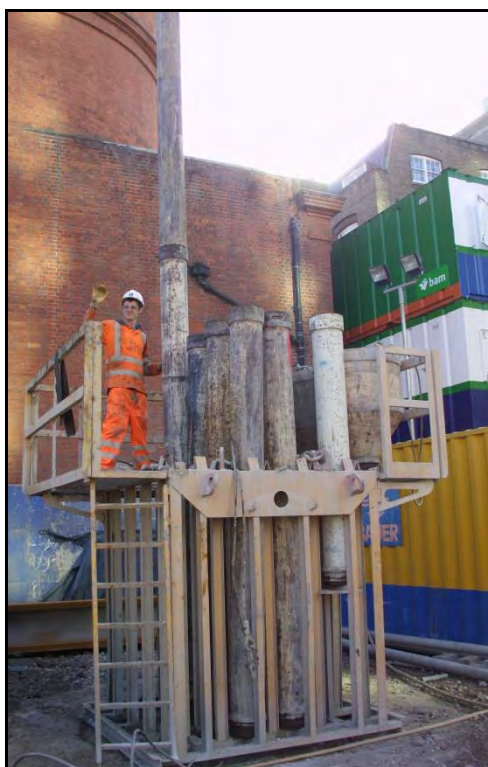
Figure 9: Photo of tremie string assembly
