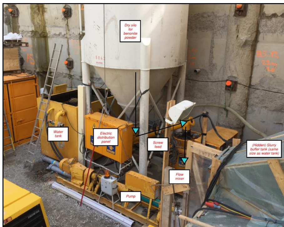
Figure 5: Typical slurry mixing setup
