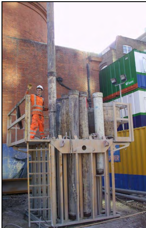
Figure 9: Photo of tremie string assembly
