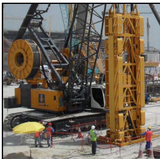
Figure 4: Cutter unit and guide frame
