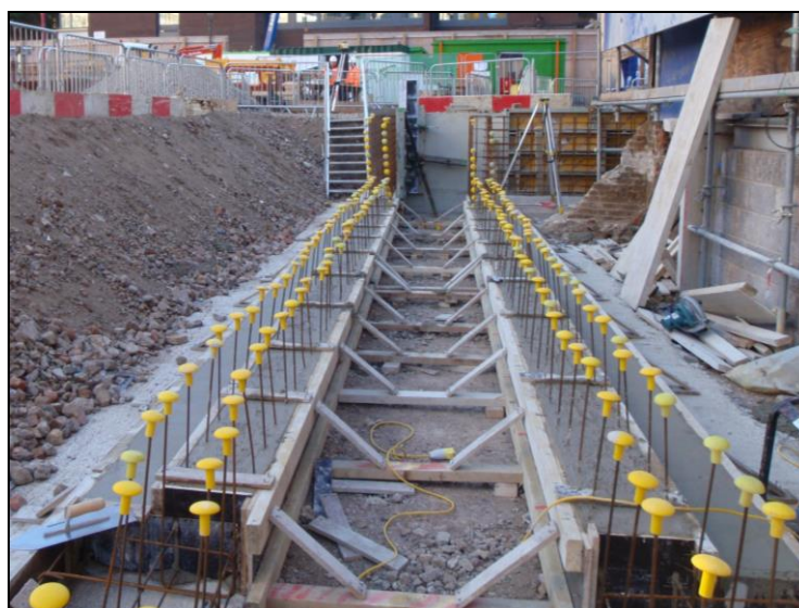
Figure 3: Construction of the base
