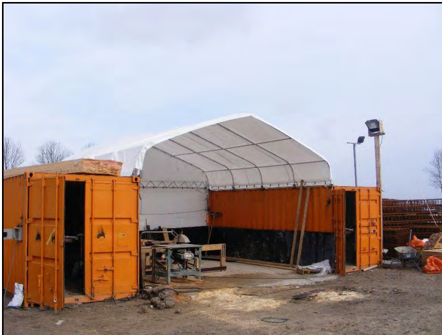
Figures 5: Example of welding tent/shelter
