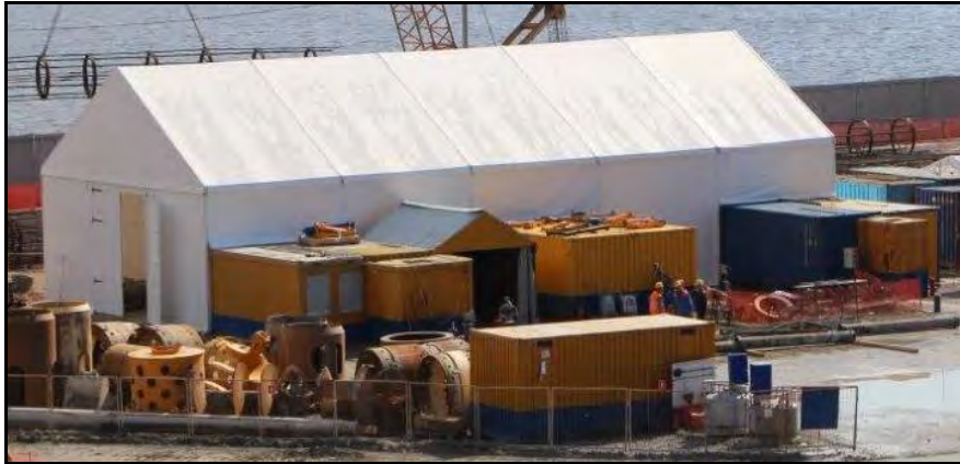
Figures 3: Example of workshop with store containers installed to the sides
