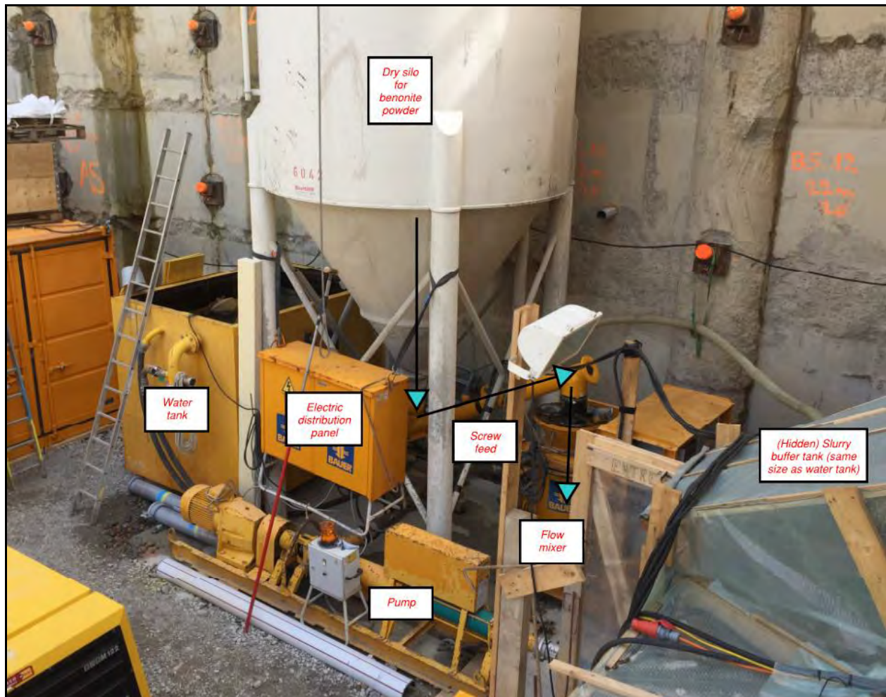
Figure 1: Typical slurry mixing setup
