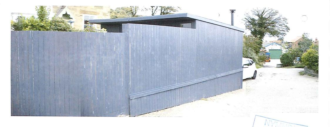
This is the existing view of the South and West Elevations from Nookfield Close. The railway sleeper wall is clad in vertical boarding and painted to match the building above, although this may make the building appear larger/taller than it is.
