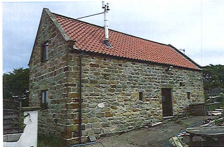
Fig. 6: View of High Mitten Cottage looking south east.
