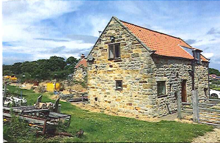
Fig. 5: View of High Mitten Cottage looking north west.
