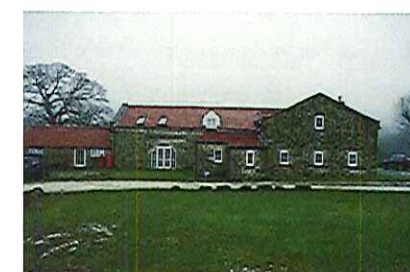
Fig. 9: View of the North elevation with lean-to kitchen extension in the centre to be removed
