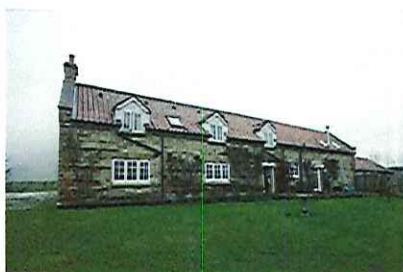
Fig. 7: View of South West / front elevation
