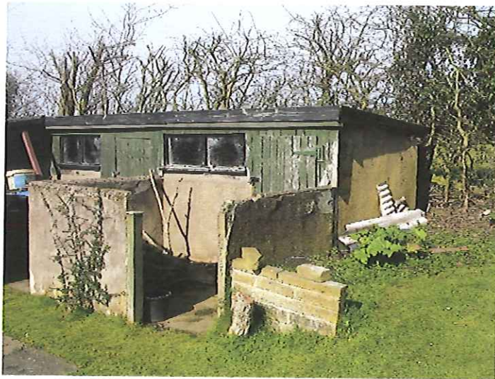
Front elevation from adjacent wall.
