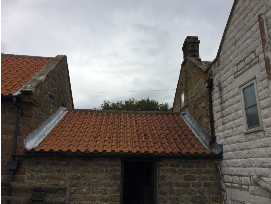
Figure 1: Existing building without the flue
