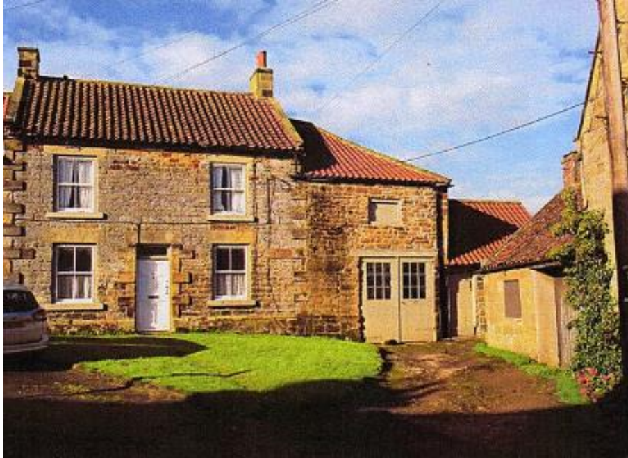
Photograph 3 – Looking South-West to the Principal Elevation of 10 South End
