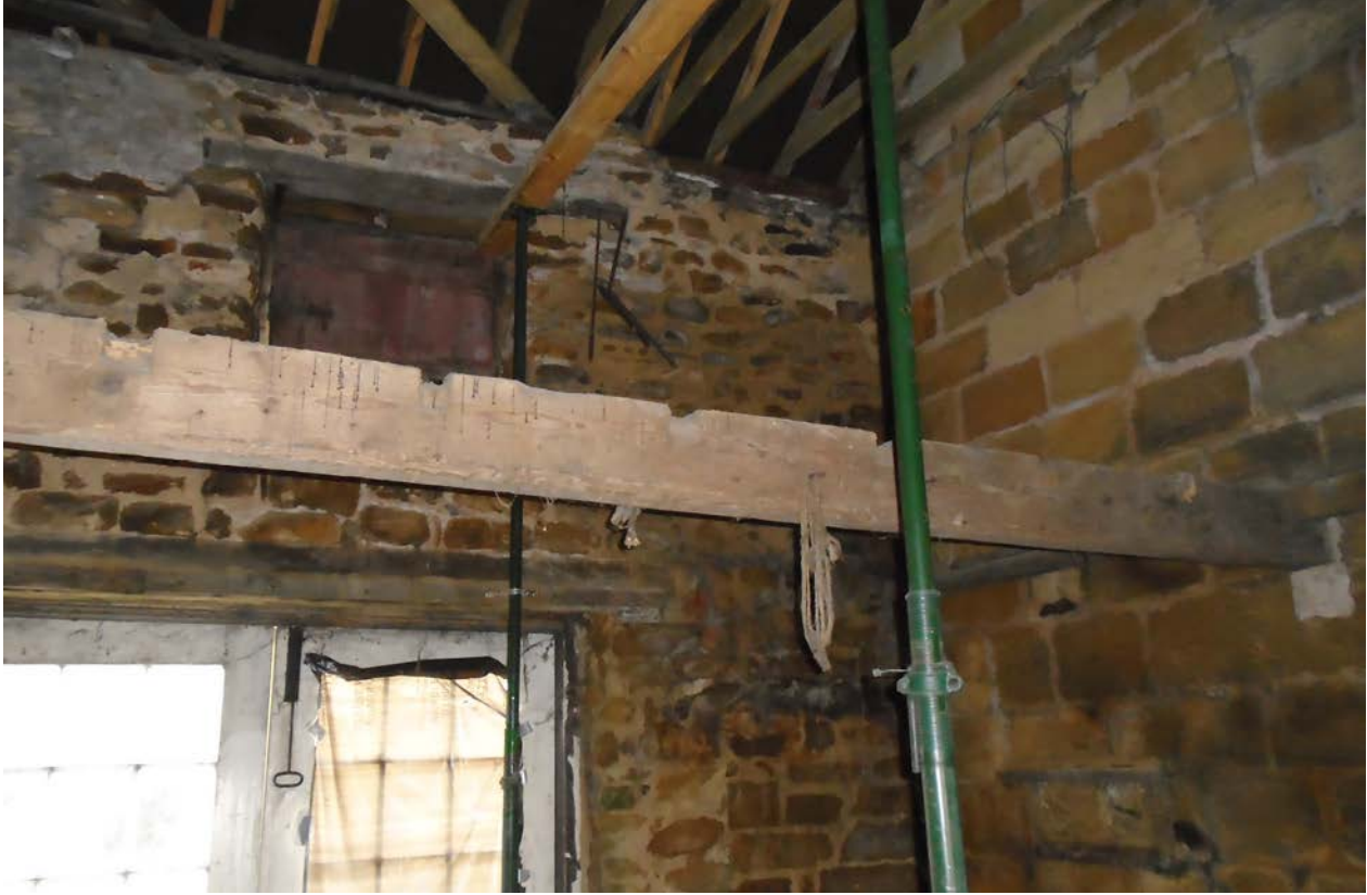
Figure 10 Main room of coach house, note blocked door and first-floor hayloft opening
