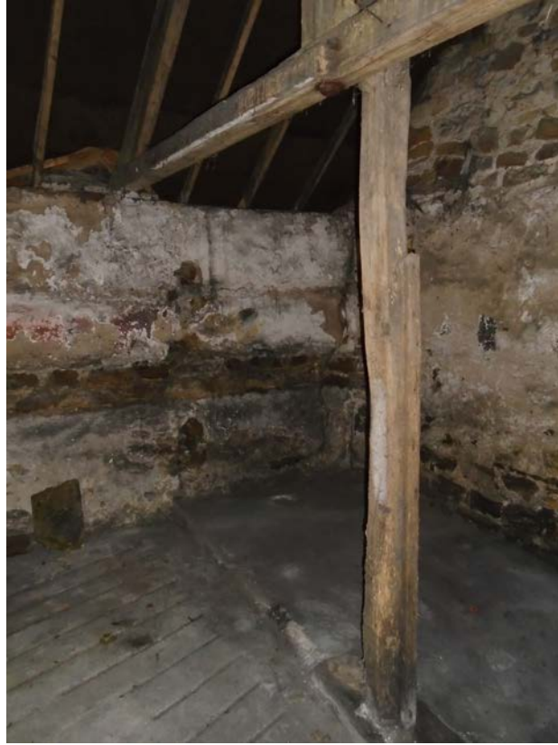
Figure 16 Concrete floor and remnants of trough
