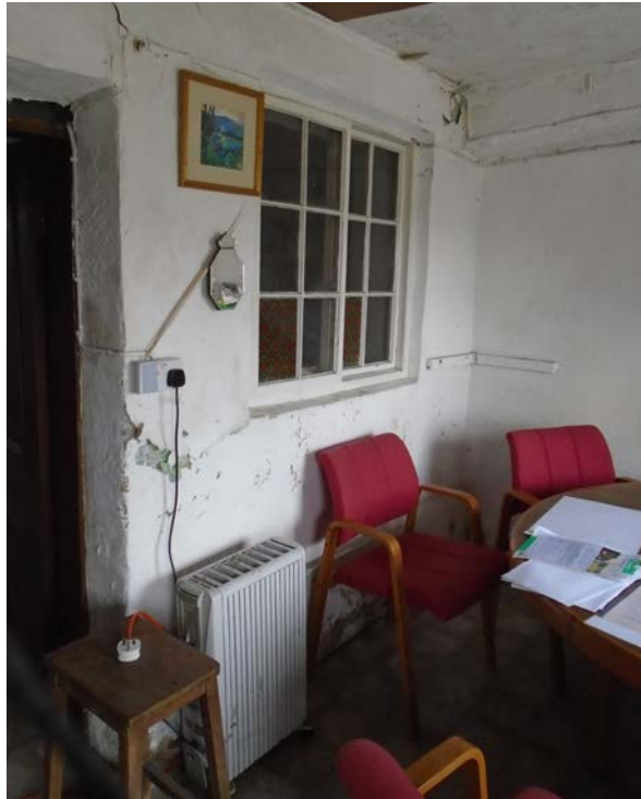
Figure 24 Original ground-floor window facing into rear extension
