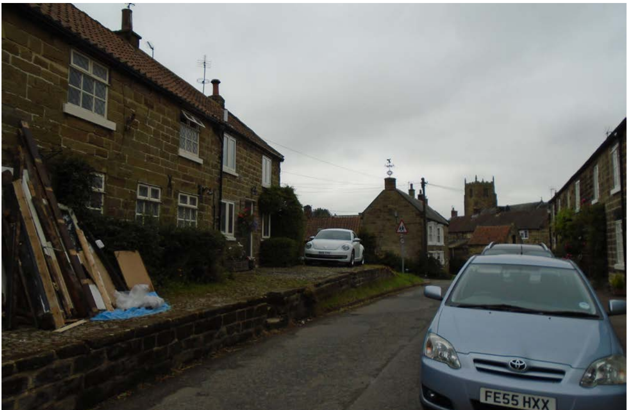
Figure 21 View along South End looking north with No. 10 obscured
