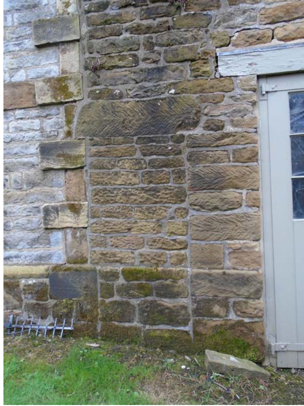
Figure 3 Detail of blocked door in coach house
