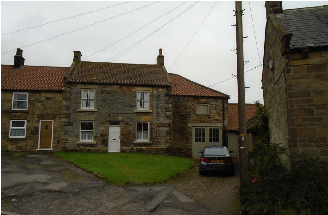
Figure 18 View from directly north-east of property
