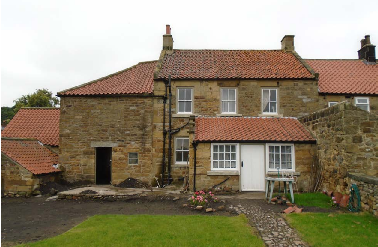
Figure 5 View looking north-east towards rear elevation
