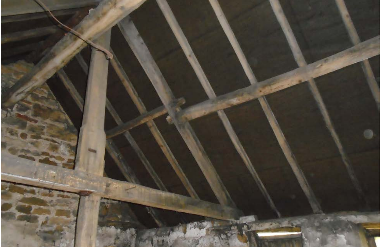
Figure 17 Mainly renewed roof structure of stable
