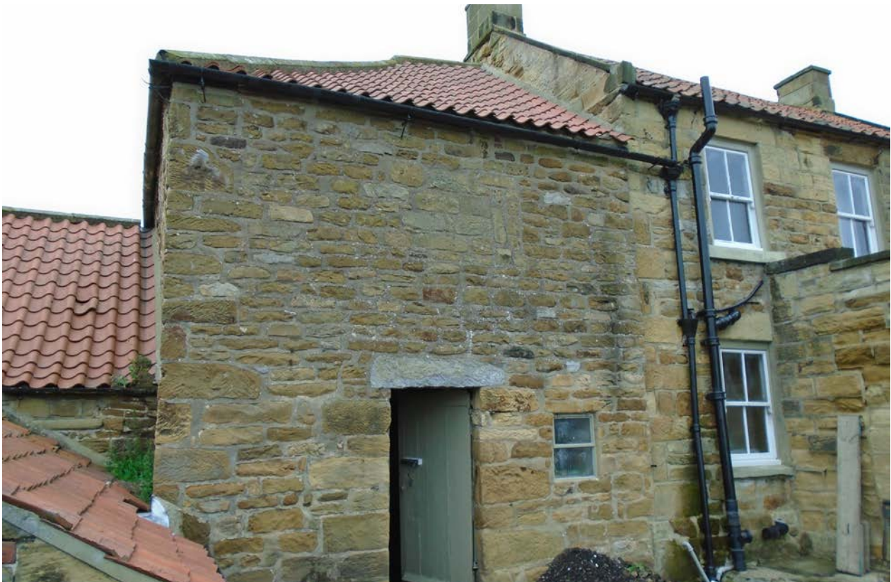
Figure 6 Detail of blocked window on rear elevation of coach house
