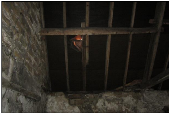
Photo 5: Internal of Block B, with rip in liner.
