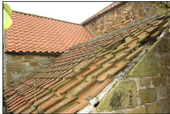
Photo 6: Roof of Block C
