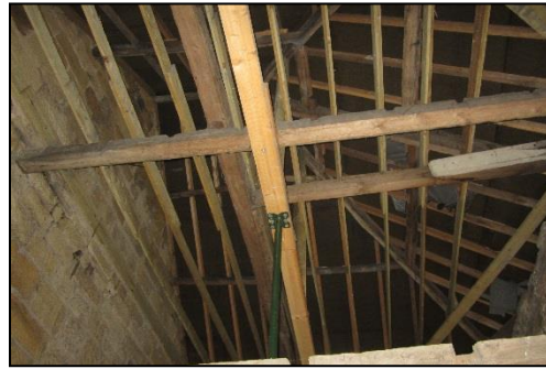
Photo 4: Internal view of roof of Block A
