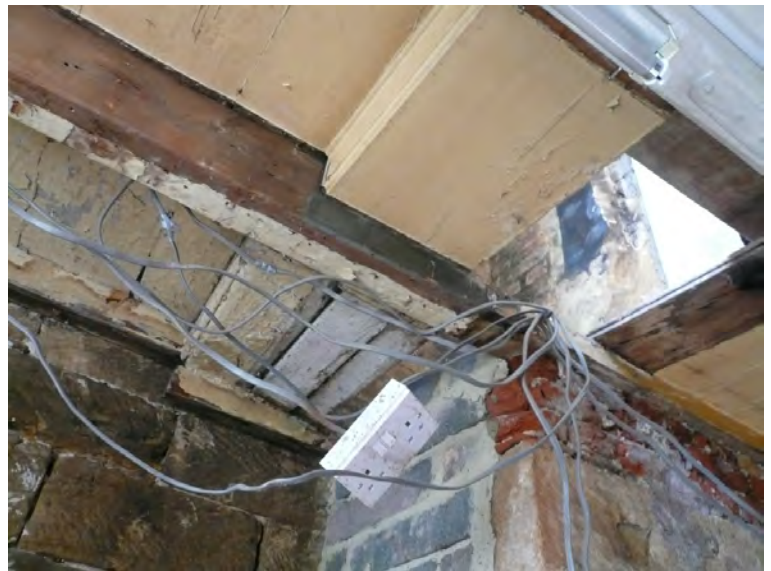
LHS fire place recess. Timber beams support masonry over.
