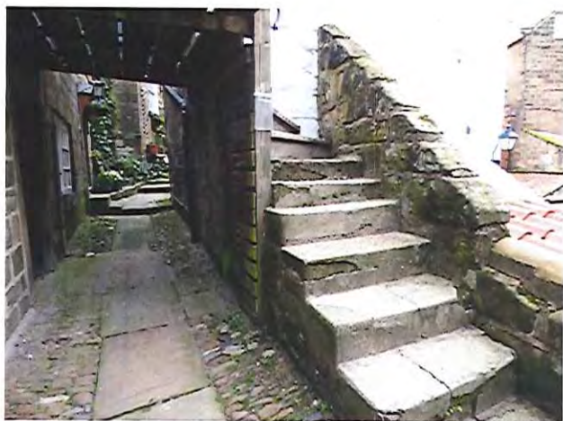
Above: Steps from St Martins row leading to the balcony.
