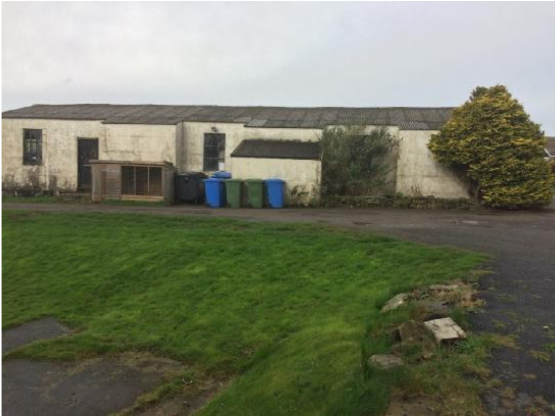
Photo 1 South East Elevation of Existing Shed
