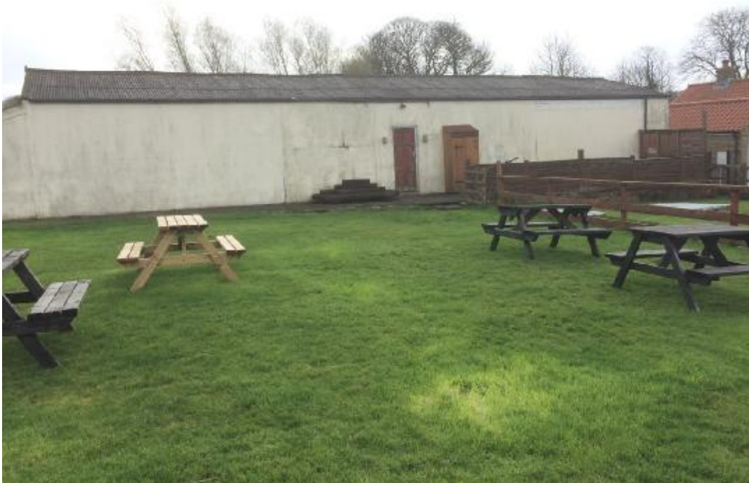
Photo 2 North West Elevation of Existing Shed
