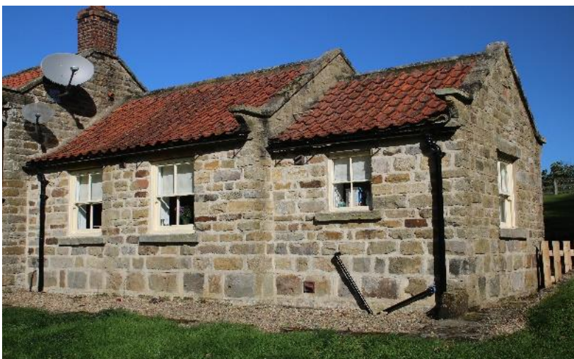
Photo 4 – W10 and W11 to be upgraded and double glazing inserted (RM01).
