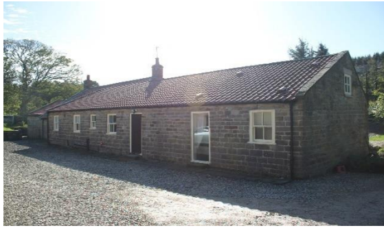
Photos 29a, 29b and 29c - Existing double-glazed windows W01, W02 and W19 (high level) to be upgraded and double glazing inserted. Existing single glazed window W18 to be replaced with timber sliding sash with double glazing (RM14).
