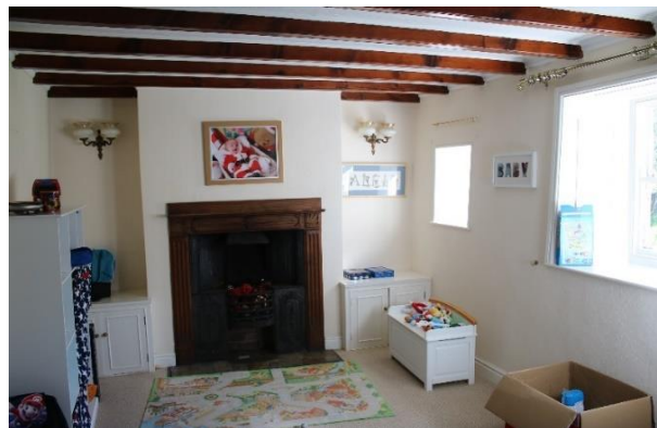
Photo 11 – Existing fireplace to be retained. Timber fire surround to be removed (RM04).
