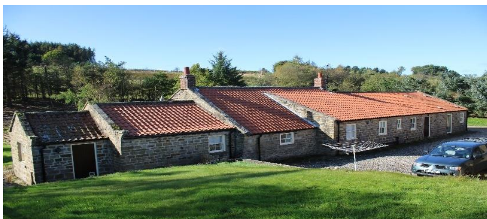
Fig. 2. Providence Heath, Cloughton – rear elevation as it is today
