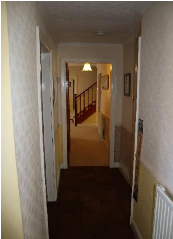
Photo 15 - Existing fully glazed door, frame and small section of surrounding wall to be removed (RM05).
