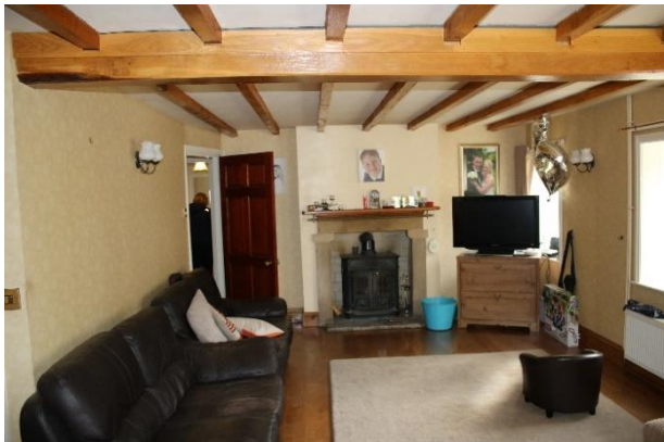
Photos 24a, 24b and 24c - Existing fireplace to be removed and replaced with new more sympathetic simple brick fireplace with timber mantle and new wood burner (see suggested example below) (RM10).
