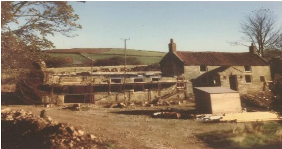
Fig. 7. Providence Heath, Cloughton – during construction – 1985 approx.
