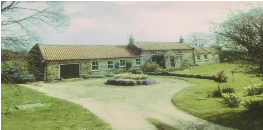
Fig. 10. Providence Heath, Cloughton – post construction – 1985/90 approx.
