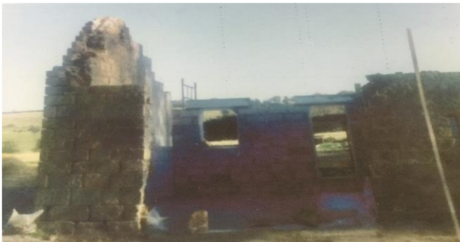
Fig. 9. Providence Heath, Cloughton – during construction – 1985 approx.
