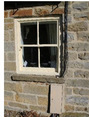
Photos 25a and 25b - Existing single glazed window (labelled D3) and masonry below carefully removed. New full height double glazed window unit to be inserted (RM10).
