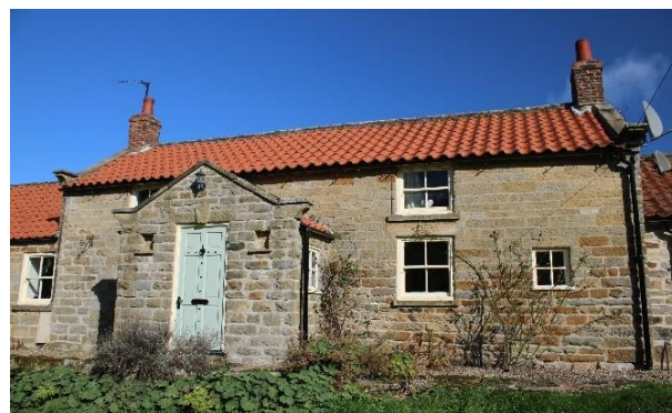
Photo 12 – Existing windows W14, W15 and W20 and W21 to be replaced on an exact like for like basis exclu internal horn detail (RM04).
