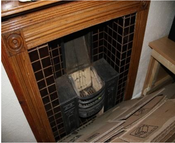
Photo 16 - Existing fireplace to be retained. Non-original timber fire surround to be removed and replaced (RM06).
