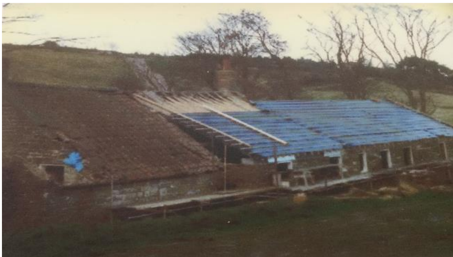
Fig. 8. Providence Heath, Cloughton – during construction – 1985 approx.
