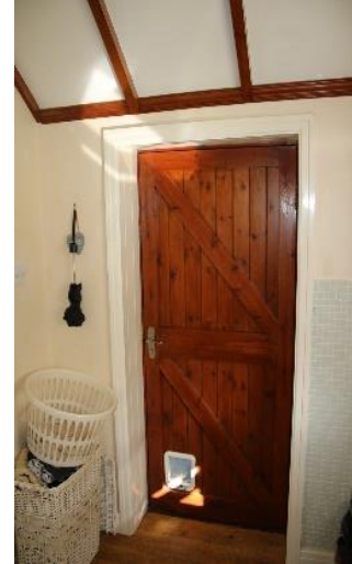
Photo 2 – Inside doorway to be blocked up (RM01).
