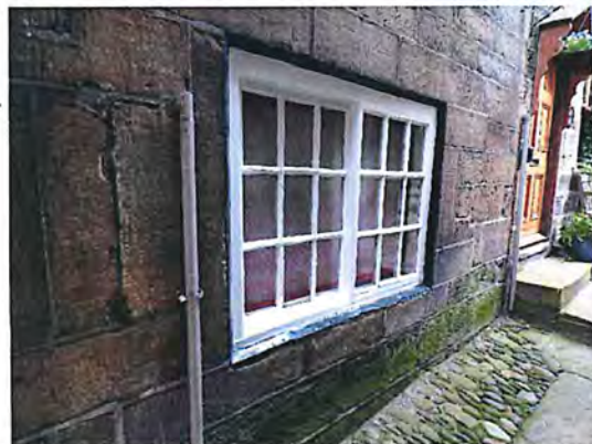
W1 – Existing Yorkshire sliding sash window Has been repaired and redecorated numerous times, and now it is proposed to replace the Existing window with a traditional style double glazed slim conservation window
