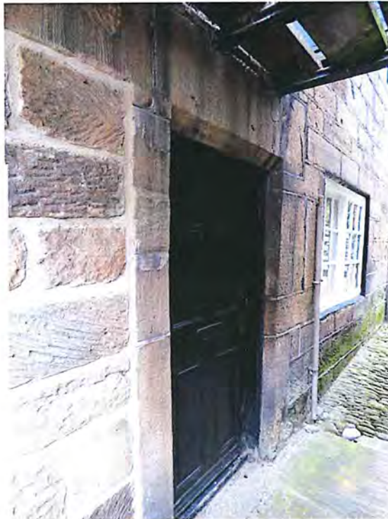
W1 – Existing Yorkshire sliding sash window Has been repaired and redecorated numerous times, and now it is proposed to replace the Existing window with a traditional style double glazed slim conservation window
