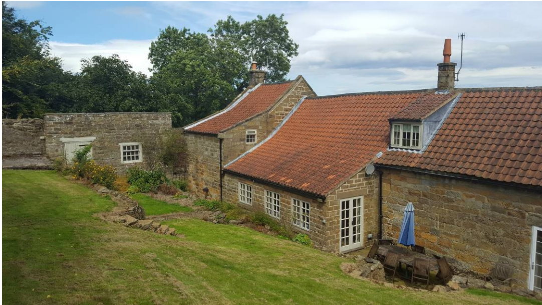
View of Existing Farm House Looking North West
