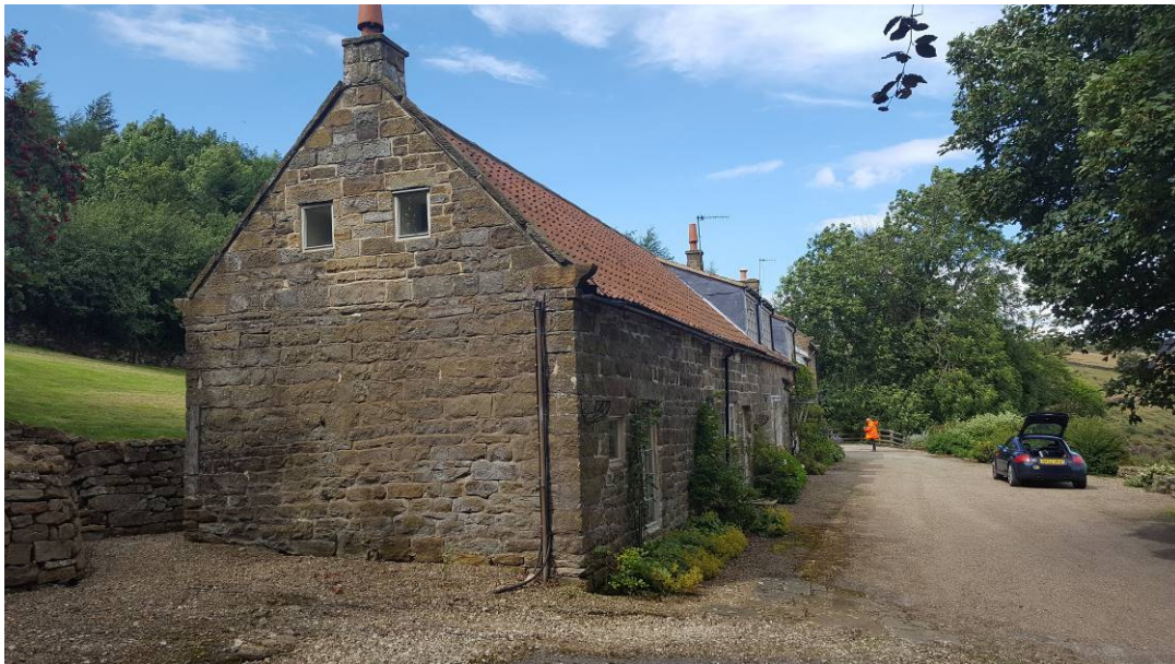
View of Existing Farm House Looking North West
