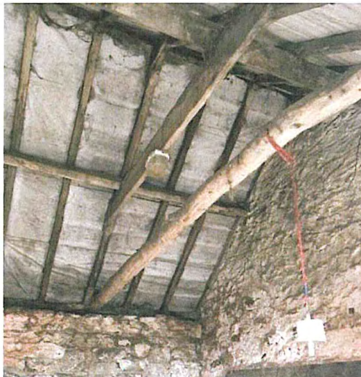
Plate 6 –roof structure of the barn
