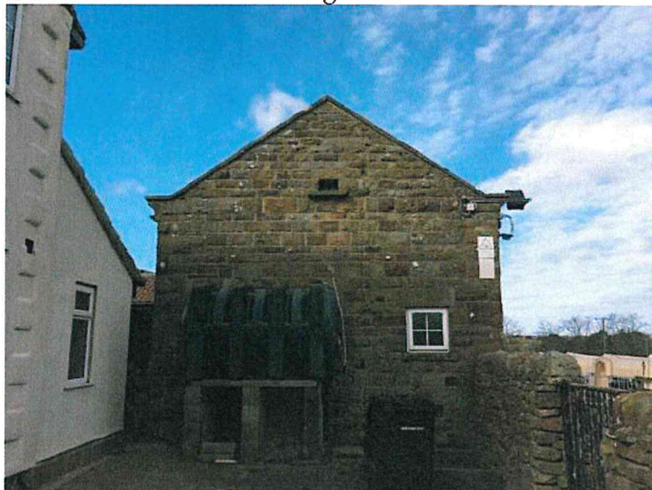
Plate 3 – South gable of the barn.
