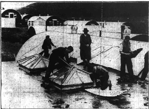
PREPARING THEIR TRAINING CENTRE.—Some of the first men at the Allerston Instructional Centre erecting huts in the camp, to be officially opened shortly.
