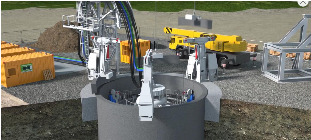
Figure 4: Lifting precast rings into position
