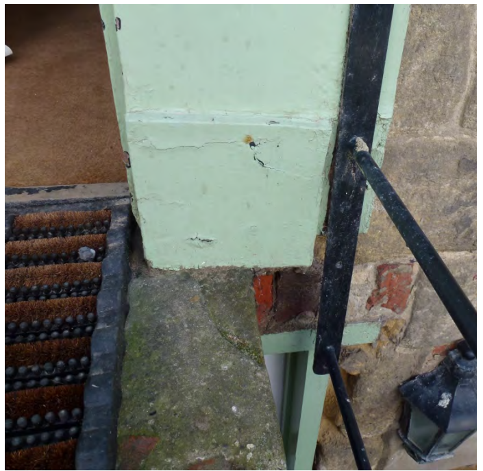
Photo 10. Front Door surround RHS.
