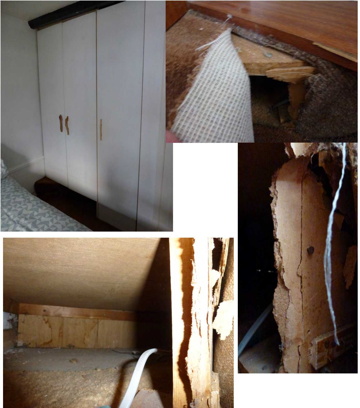
Top rhs. Internal view at base
