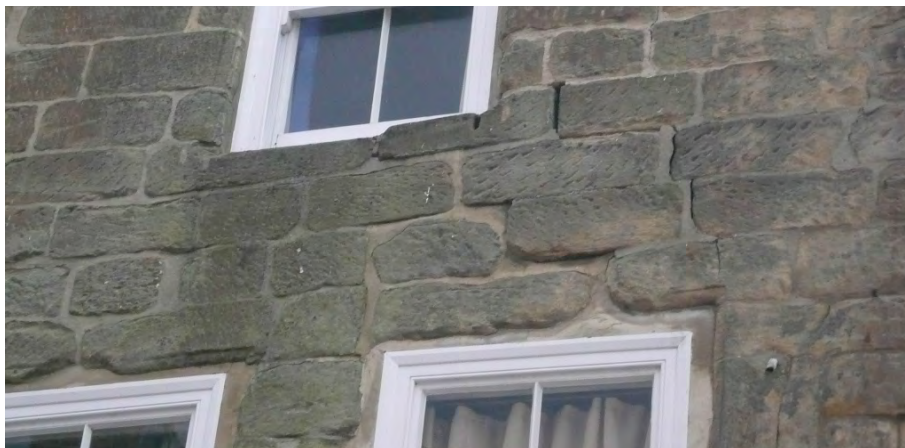
Photo 12. First Floor heads Second Floor sill.
