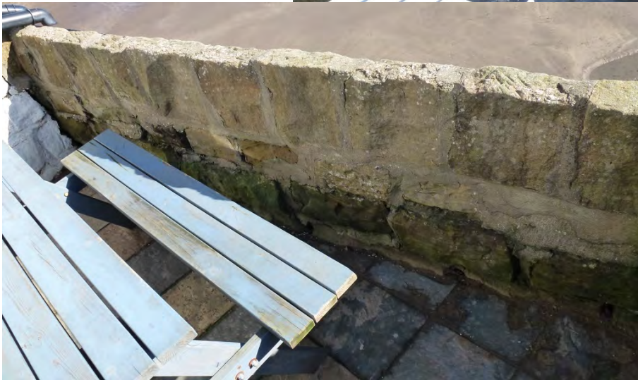
Photo 2. Terrace wall to north.
