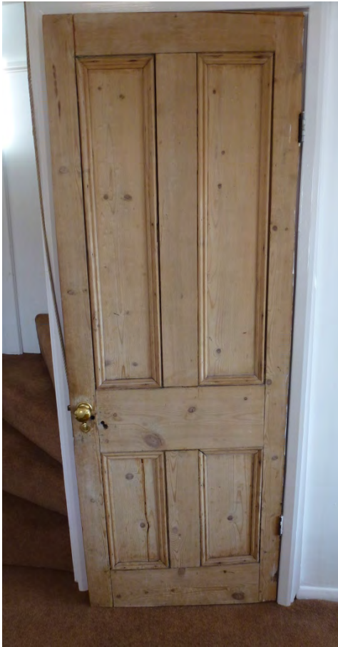
Photo 20. FFL Door to Staircase
