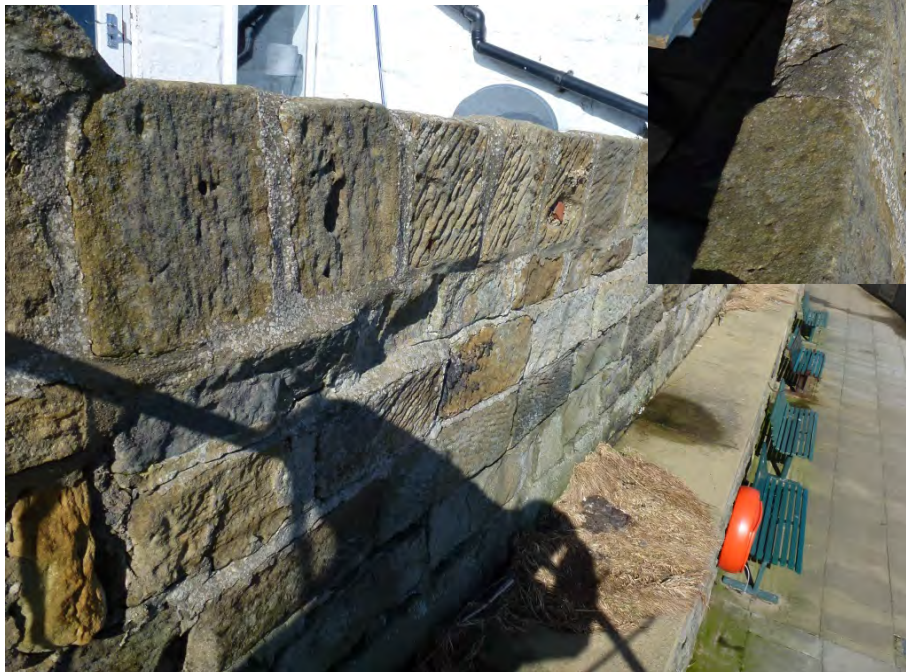
Side. Photo 4. shows weathering and high coursing
