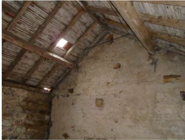
Plate 7 – Barn 2, internal roof structure
