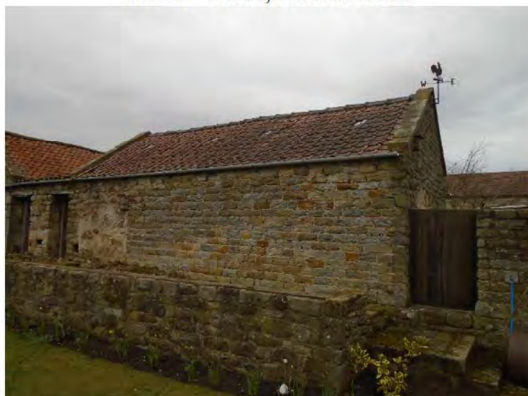
Plate 6 – Barn 2, south elevation.
