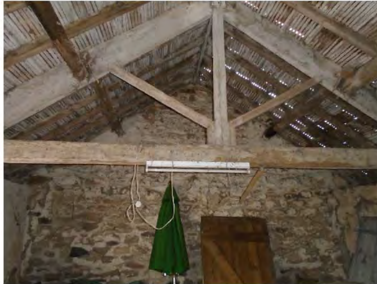
Plate 4 – Barn 1, internal roof structure.
