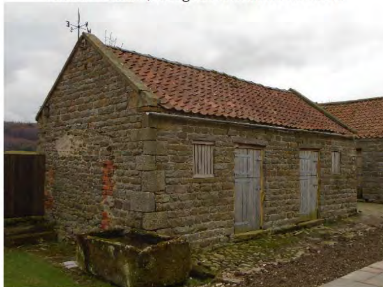
Plate 5 – Barn 2, east gable and north elevation.
