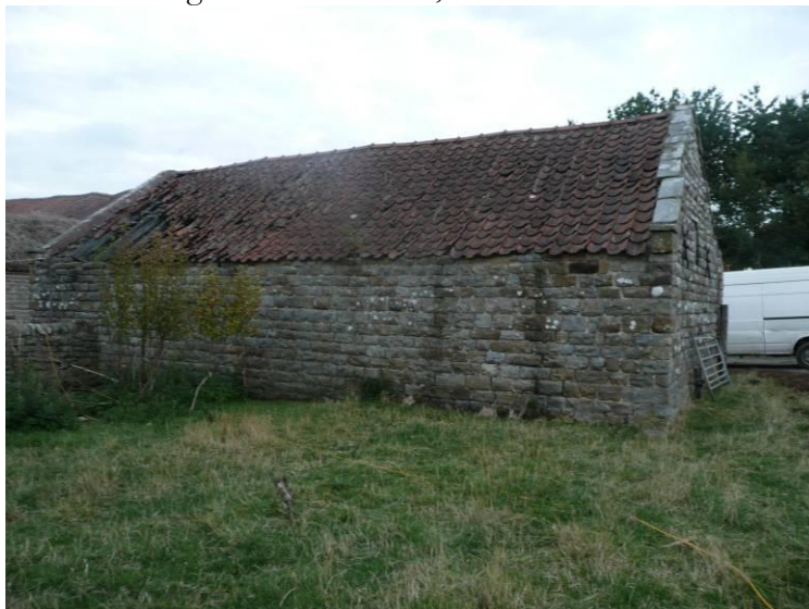
Figure 3 – Cart shed, south elevation.
