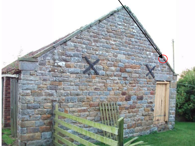
Figure 4 – Common pipistrelle roost 1, west gable of cart shed.
