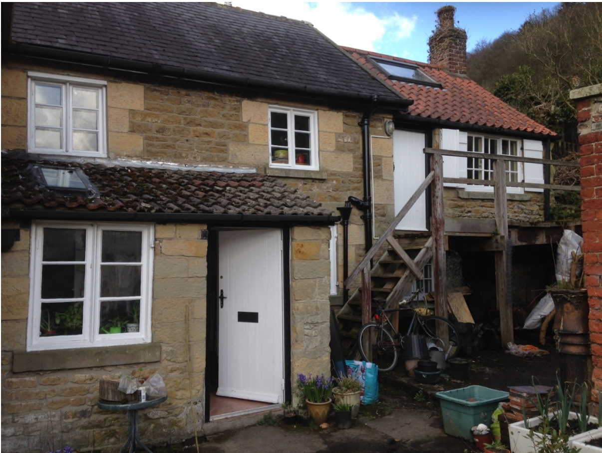
Area of proposed extension with late Victorian addition on left.
