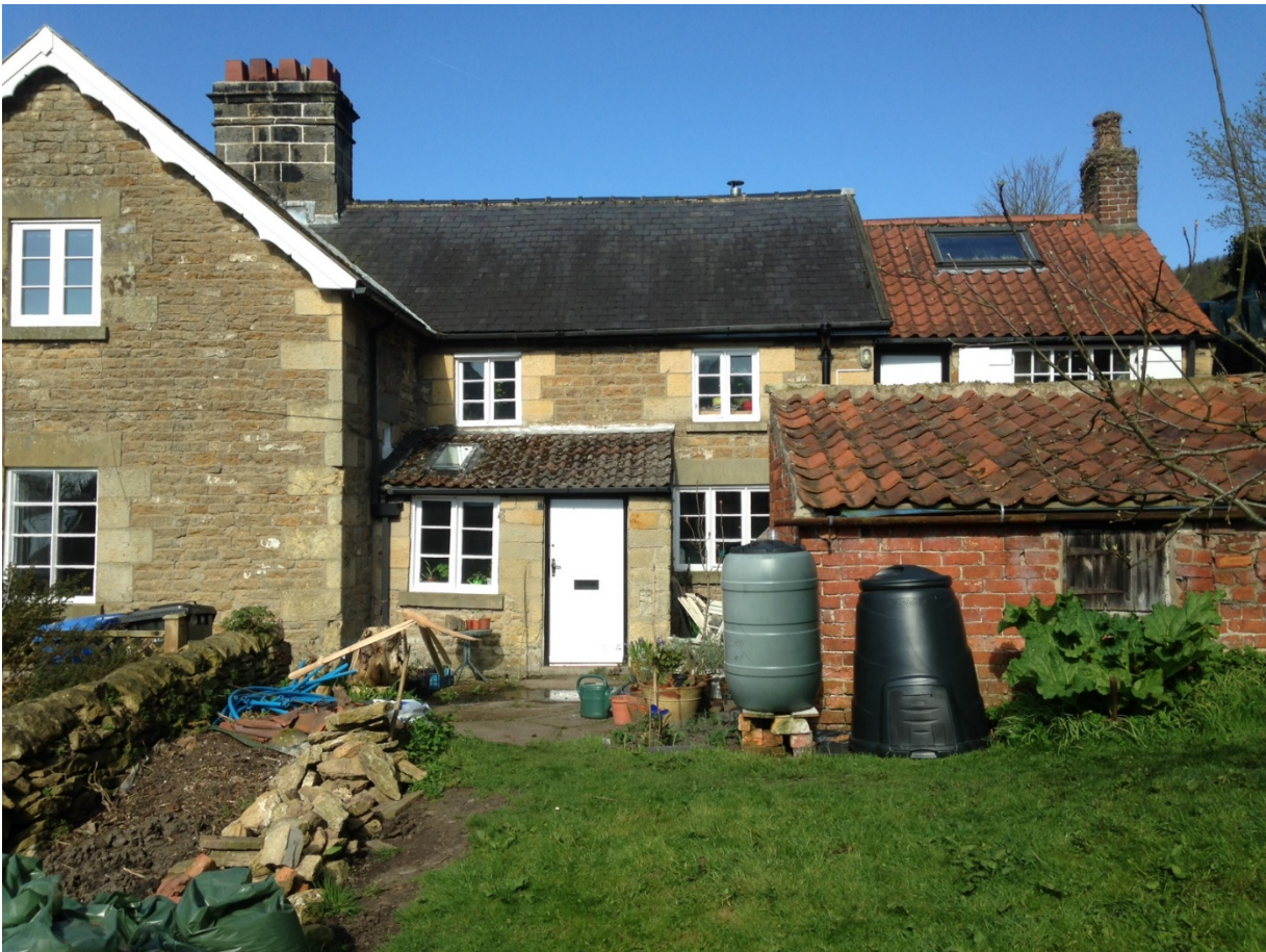
View of eastern elevation. Area of proposed extension partly obscured by pigsty and water butt.
