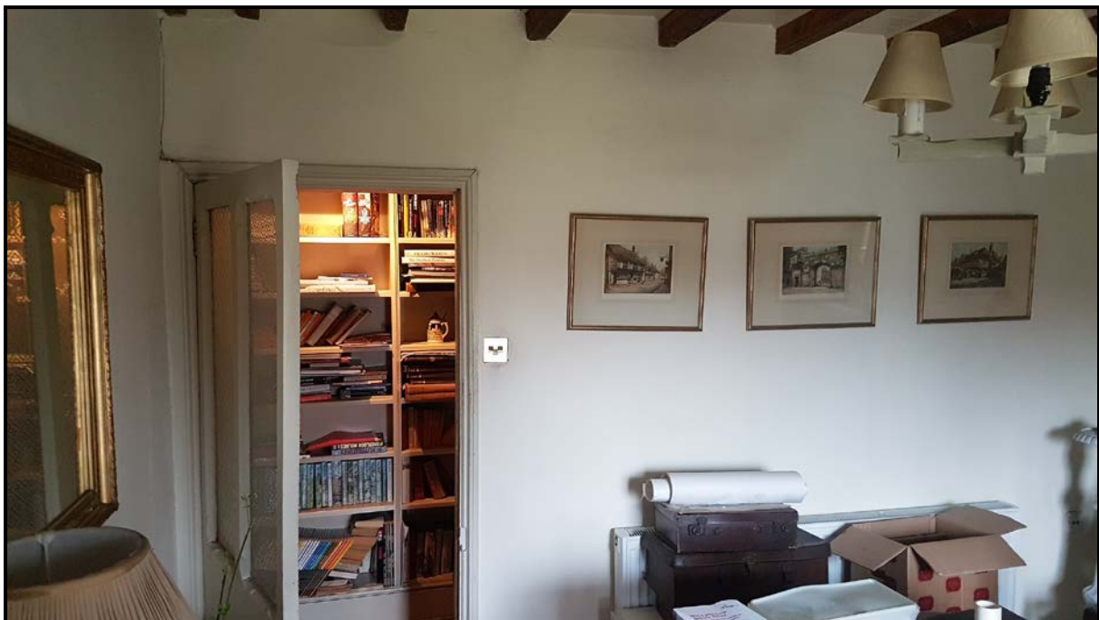
Photo 8: Dividing wall between existing dining room and library that is proposed to be removed.
