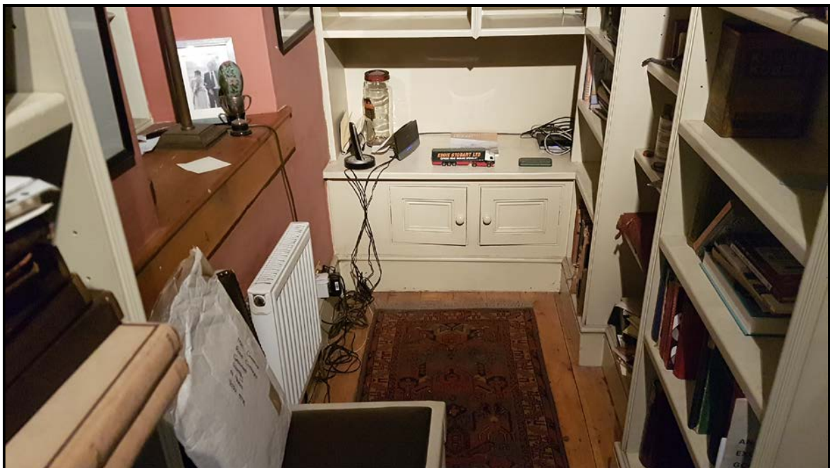
Photo 6: Library area in section divided off from existing dining room. Very dark space created.
