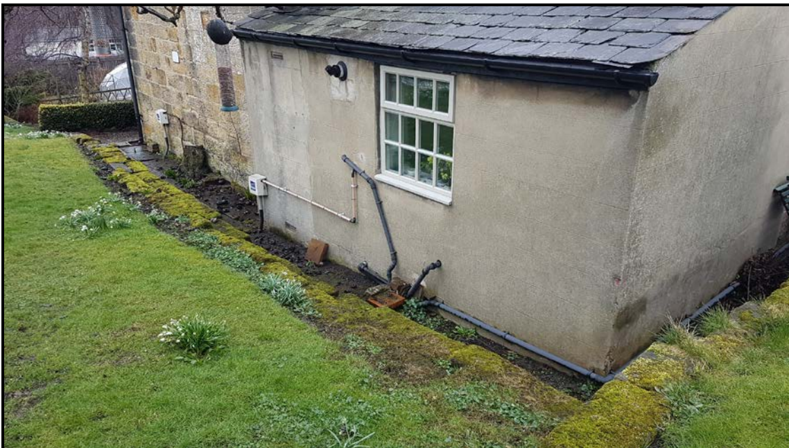
Photo 4: South side showing utility.
