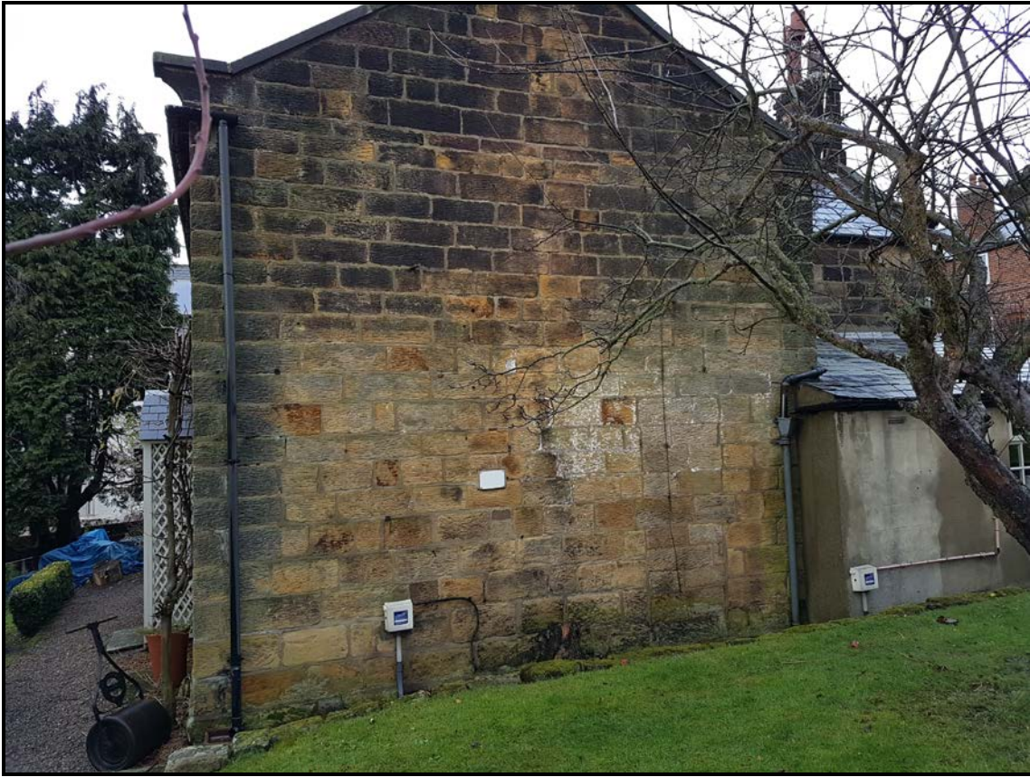
Photo 3: South side elevation.
