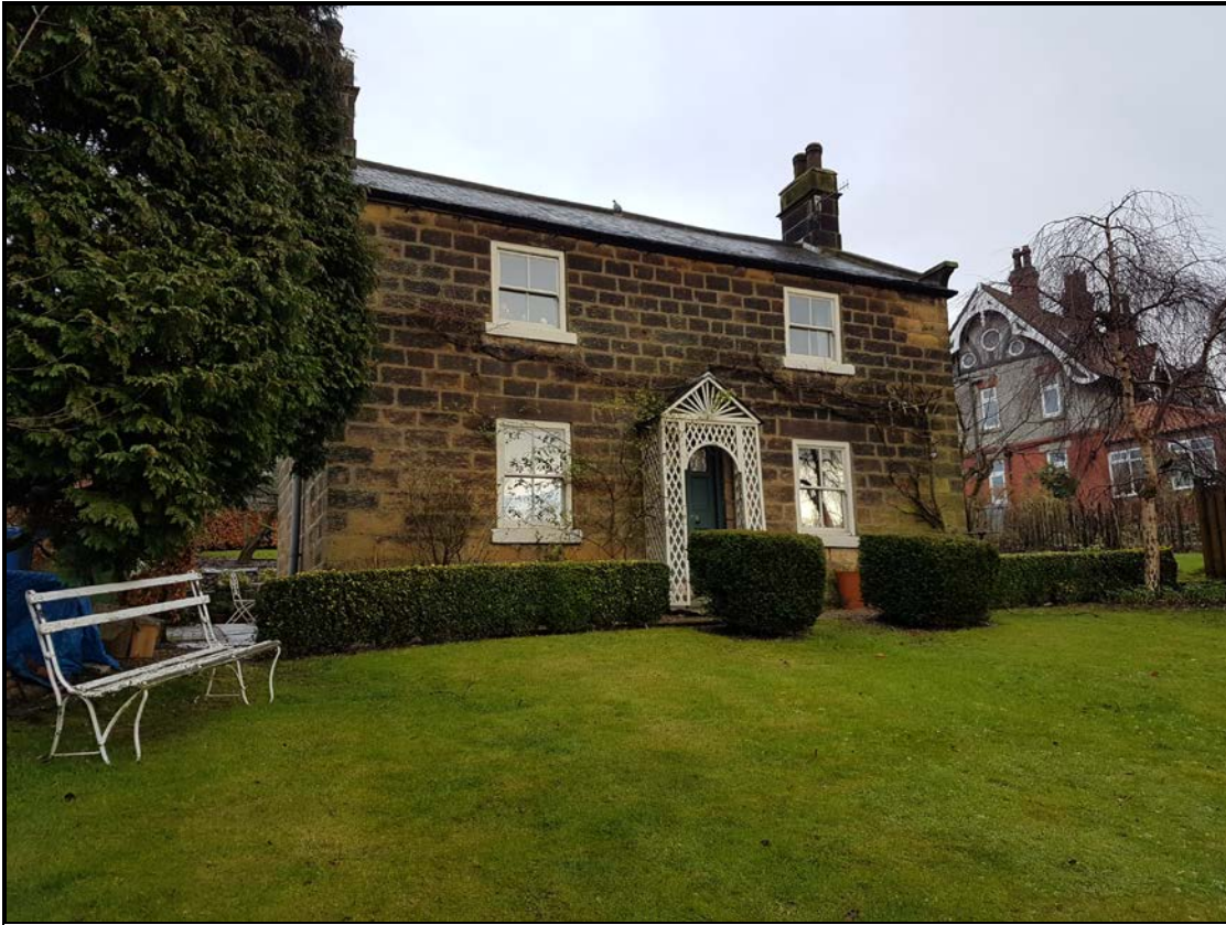
Photo 1: Principal elevation facing the railway line (West Elevation).
