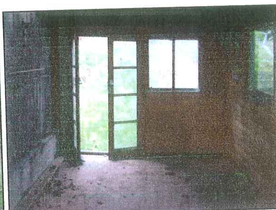
Fig. 11 Shed, interior east section
