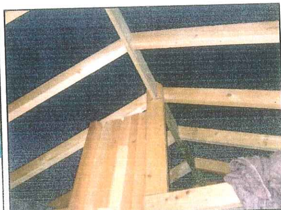
Fig. 13 Interior of garage roof
