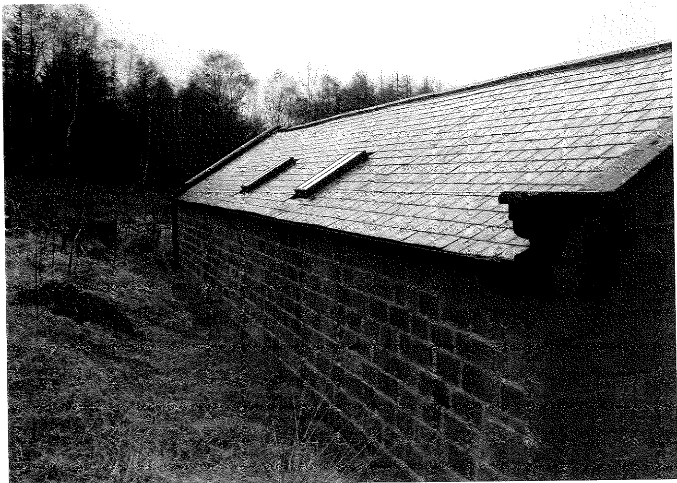
Rear roof lights-contextual setting
