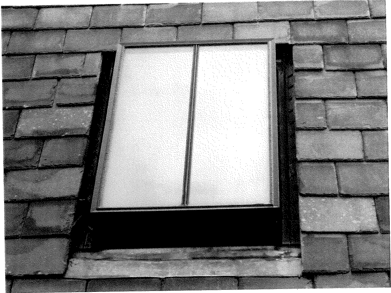
Roof lights in rear roof slope-close up.
