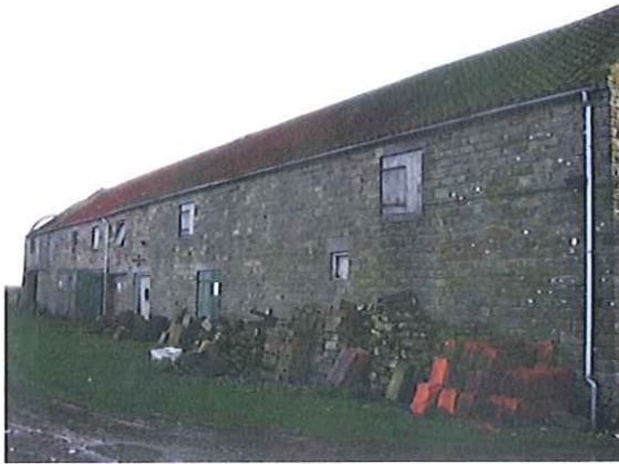
Photo 4 Northern exterior wall of areas 2,11,10,1.
