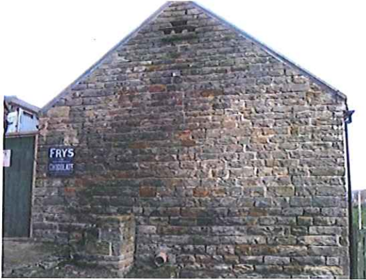
Photo 7 Gable end wall of area 4; note dove cote access
