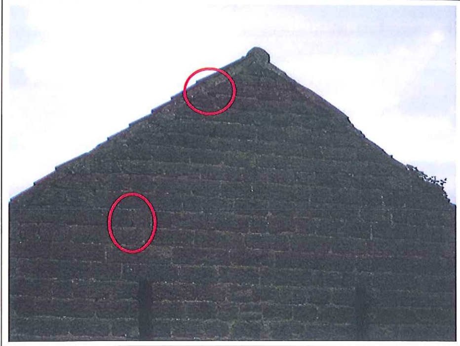
Photo 1: Access points in building 5
