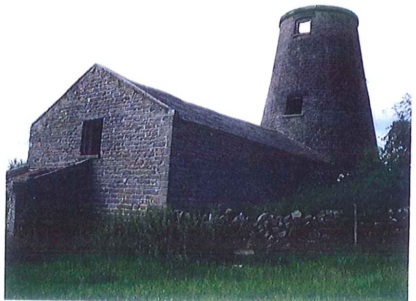
VIEW FROM NORTH EAST
