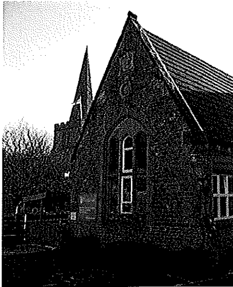
Photo 3. Original building frontage
