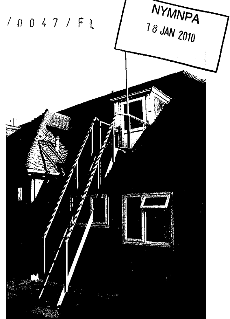
Existing second floor escape stair
