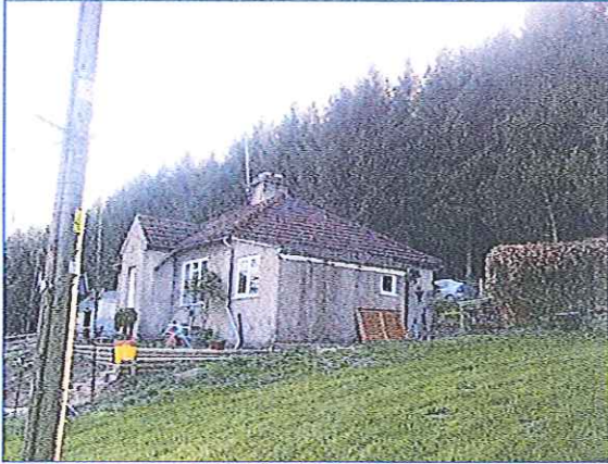
Photo 1. Bungalow from the north-east
