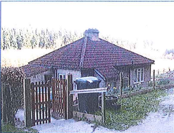
Photo 2. Bungalow from the north-west
