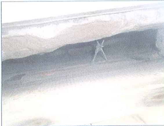
Photo 6. Cavity between inner and outer skins
