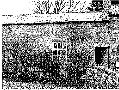
6. West facing side of building (2)
