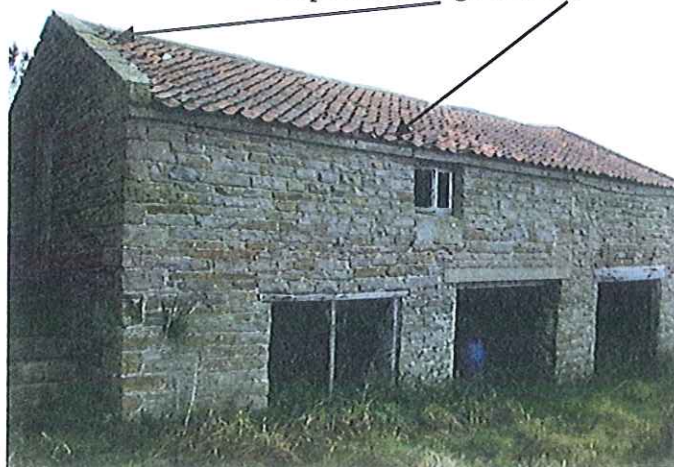
Figure 2 – Barn, north elevation.
