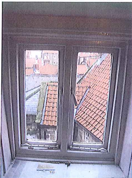
Second floor window – dormer
