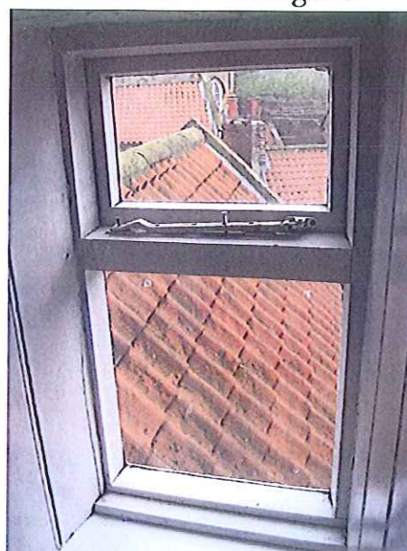
Second floor window - gable
