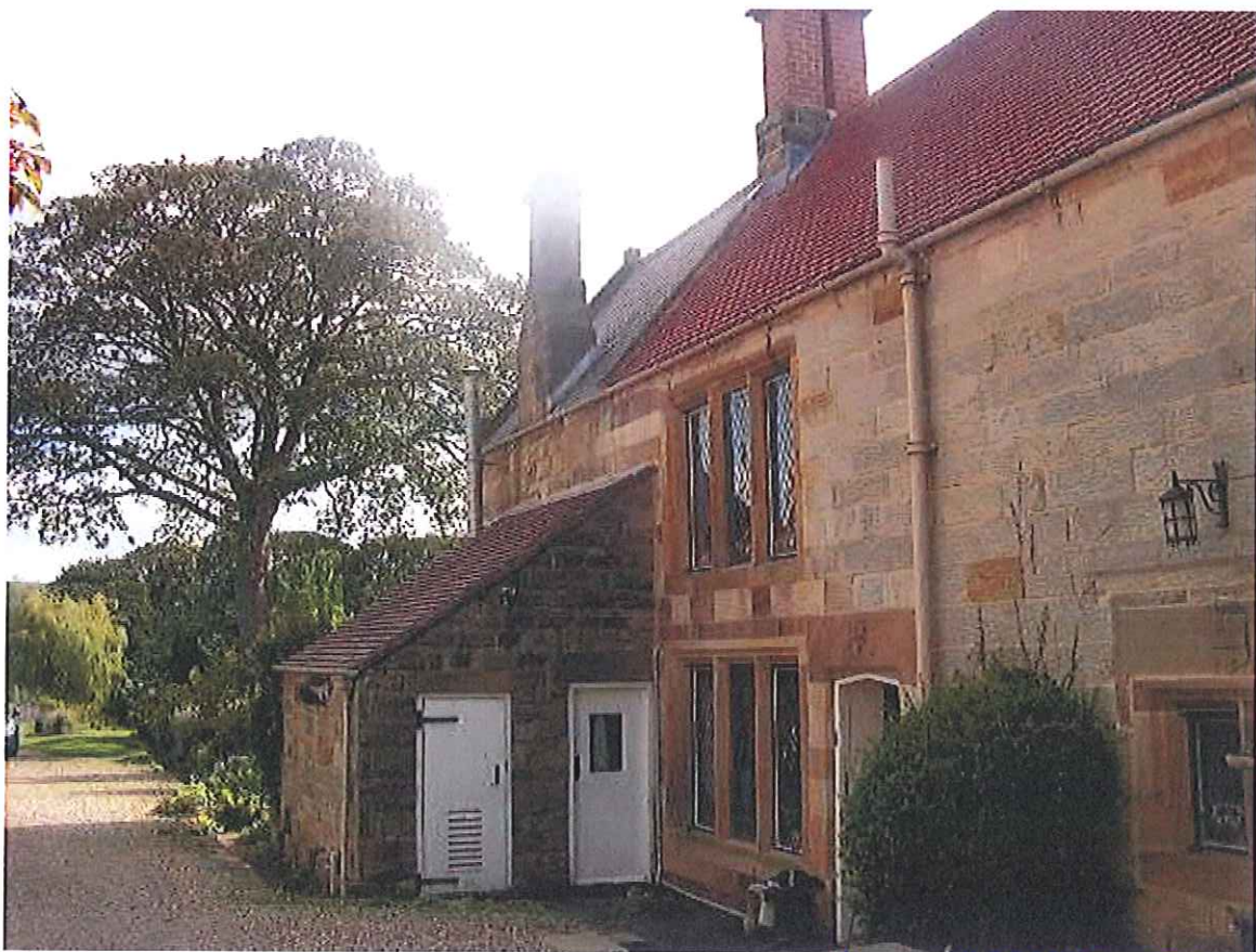
Image 01 – Utility / Boiler Room
