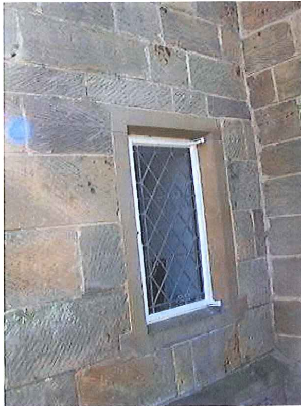
Image 06 – Existing wrought iron window
