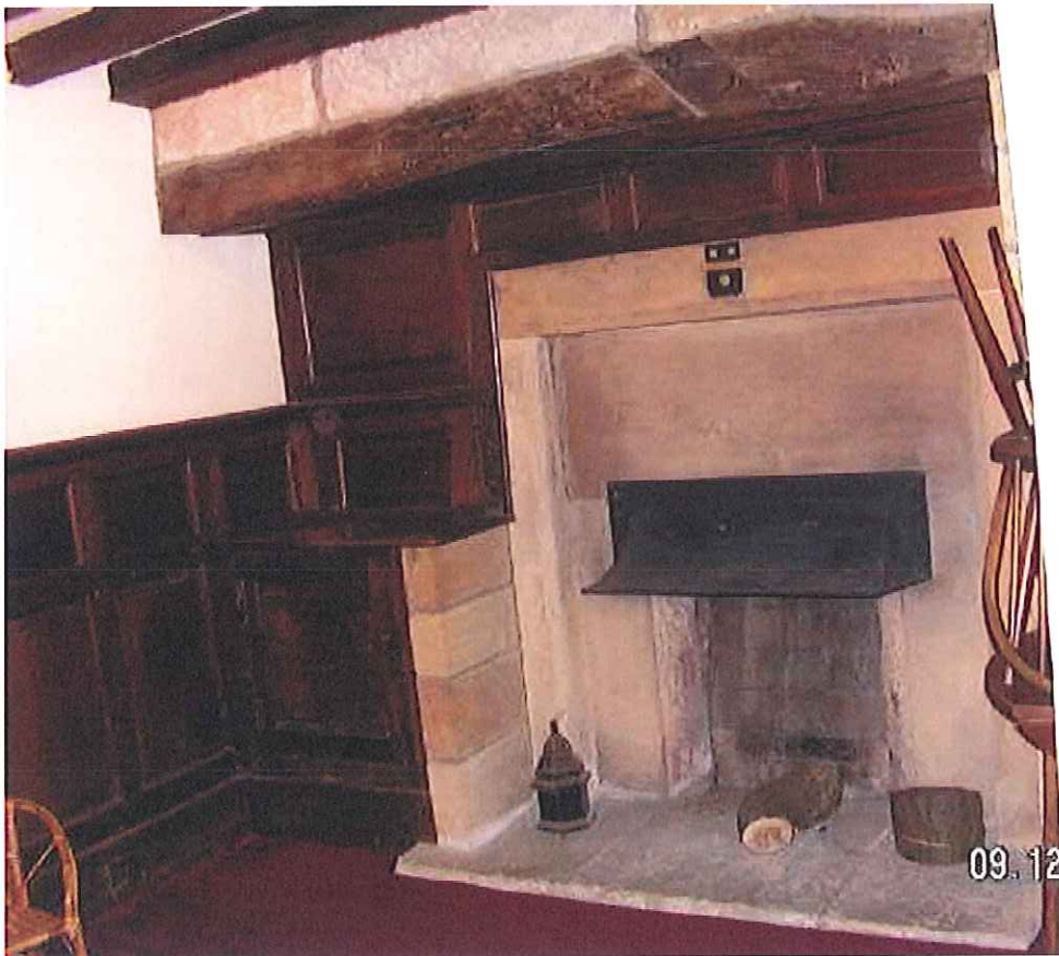
Image 02 – Panelling to be removed to the left of fireplace
