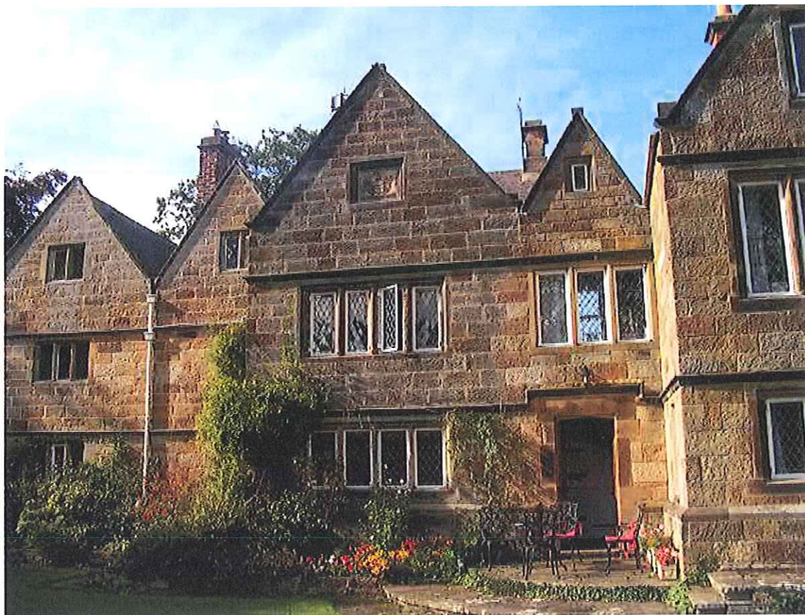
View of Thorpe Hall, Rear Elevation
