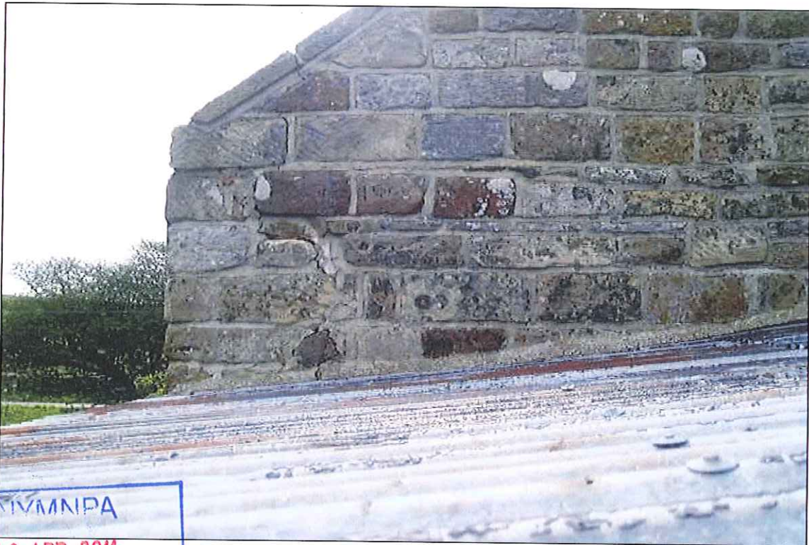
PHOTOGRAPH 8 EXISTING GARAGE, HIGH BARNS, WHITBY LAITHES
