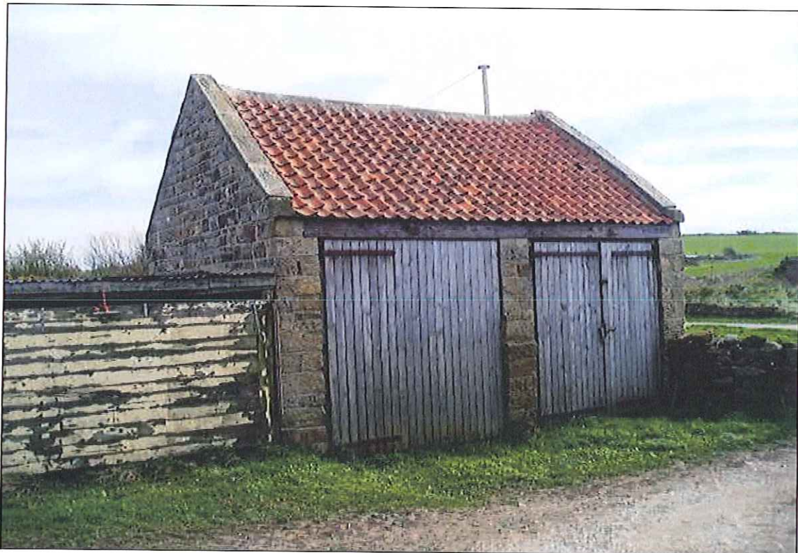
PHOTOGRAPH 1 EXISTING GARAGE, HIGH BARNS, WHITBY LAITHES
