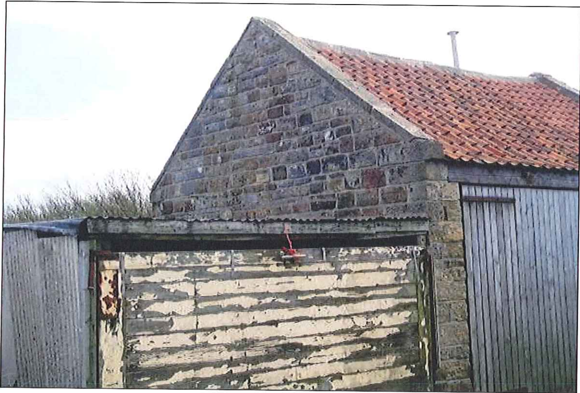
PHOTOGRAPH 7 EXISTING GARAGE, HIGH BARNS, WHITBY LAITHES
