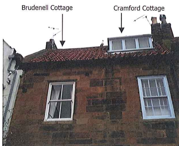
Photograph of the roof as existing
