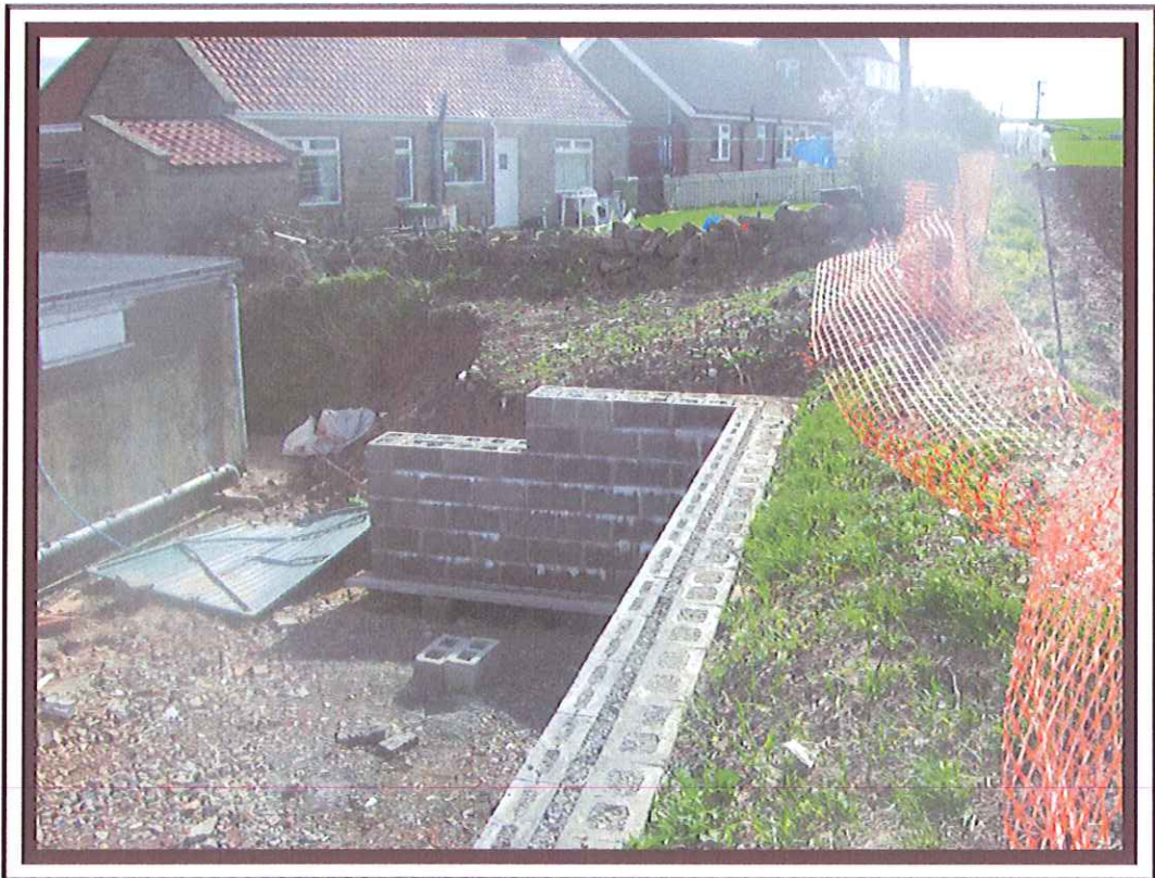
View looking south towards existing holiday accommodation from within sun terrace/patio
