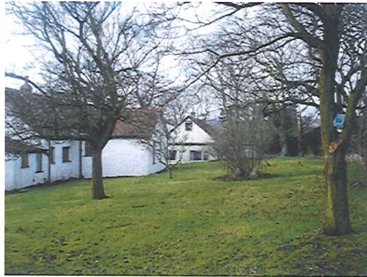
View of house from North East corner of garden
